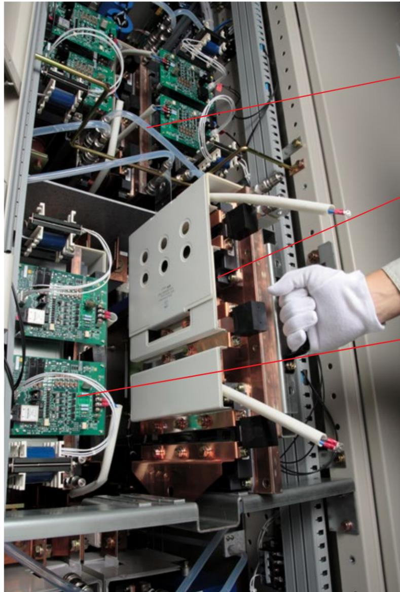
Flexible Water Cooling Tubes are easy to manage when performing maintenance.
