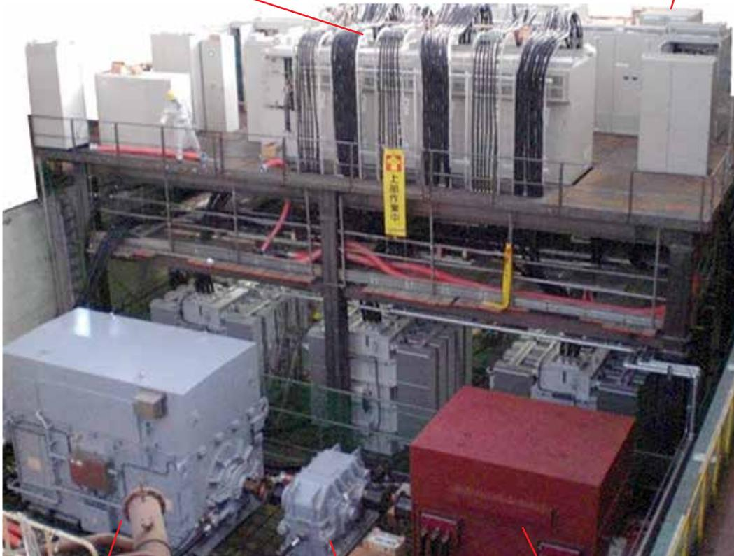
25 MW synchronous 2-pole variable speed motor, 3600 rpm
