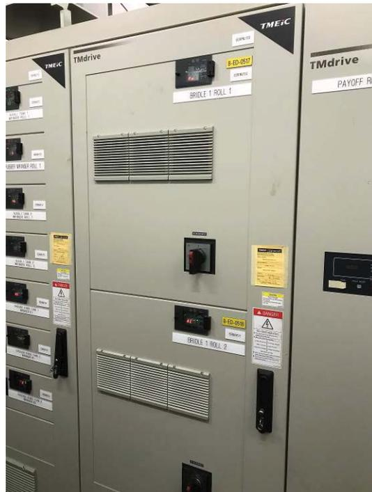
Figure 17, Entry Bridle Dual Purpose Drive
