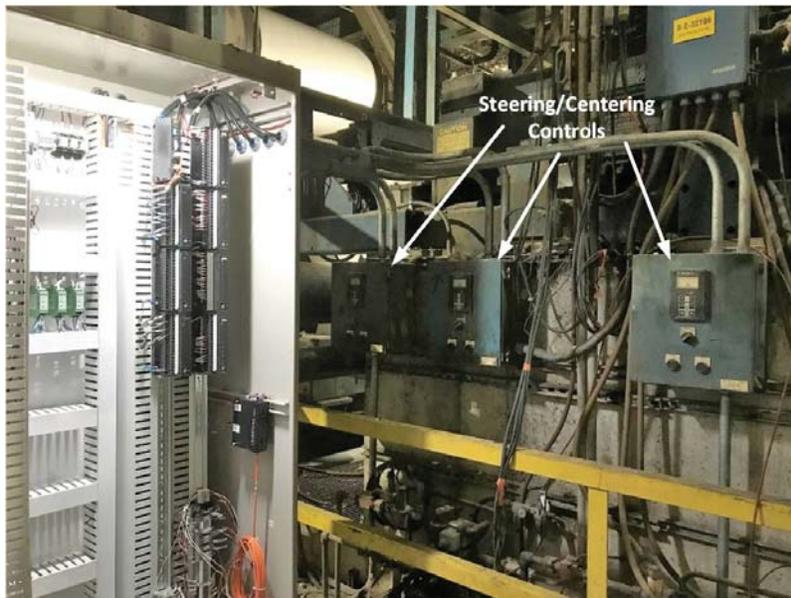
Figure 10, Steering/Centering Controllers (indicated by arrows) were replaced with new remote I/O (left) and nV Controllers. Procedures were adopted to minimize the outage time and facilitate pre-outage work prior to the shutdown. Existing wiring that was to be re-used was double tagged with both the existing wire number and the new wire number to speed and improve accuracy of wiring changes.
