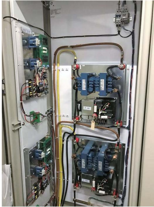
Figure 18, Aux DC panel for Dual Purpose Drive
