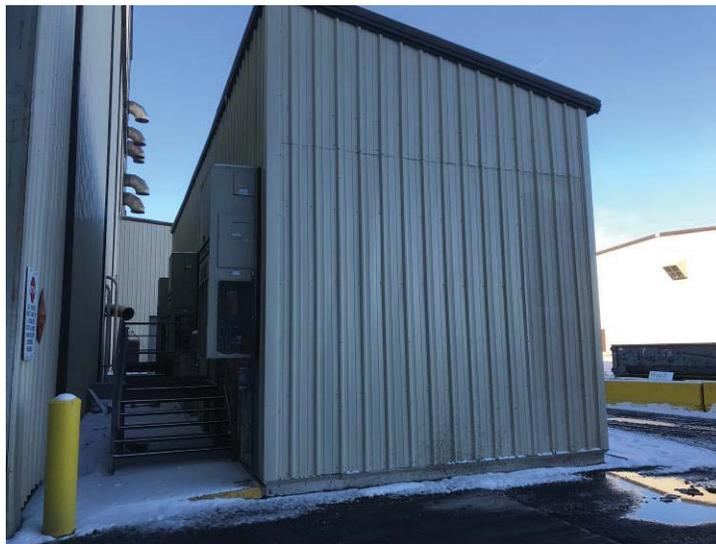
Figure 9 One of three new E-houses for new Drives and Automation Equipment
