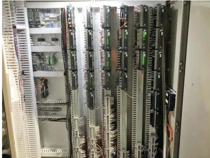
Figure 20, new nV Remote I/O
