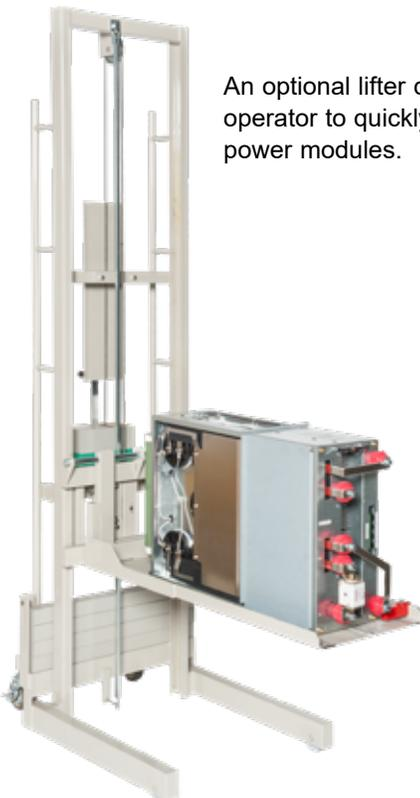
An optional lifter cart enables the operator to quickly rack-in/out the power modules.
