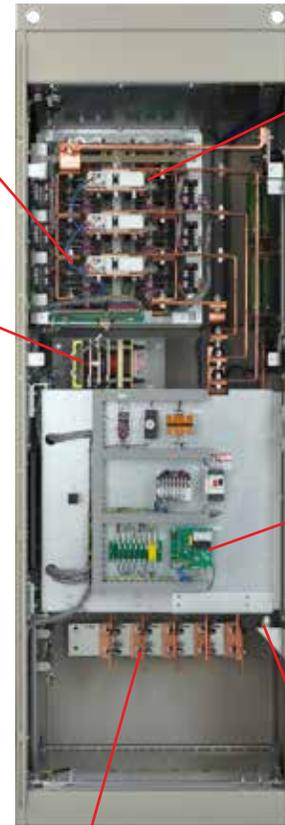
AC Leg Fuses protect power bridge from faults on the ac line
